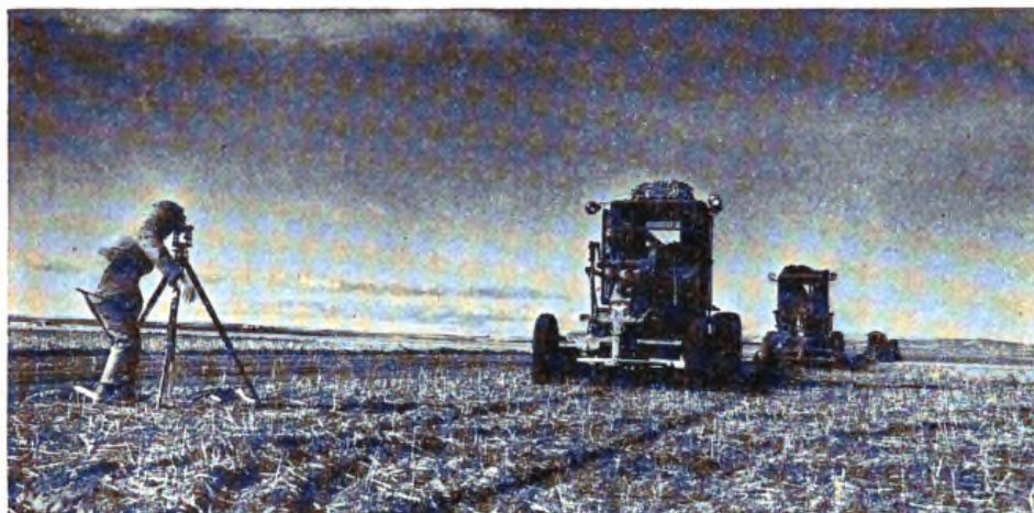
① Start of work.
